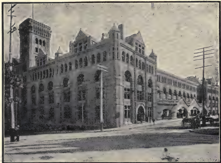
FIG. 88—Canadian Pacific Railway Windsor Station, Montreal
